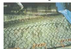
Cracked Retaining Wall
