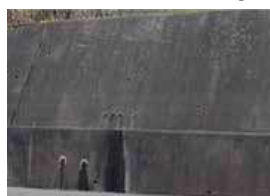
Groundwater Leakage
